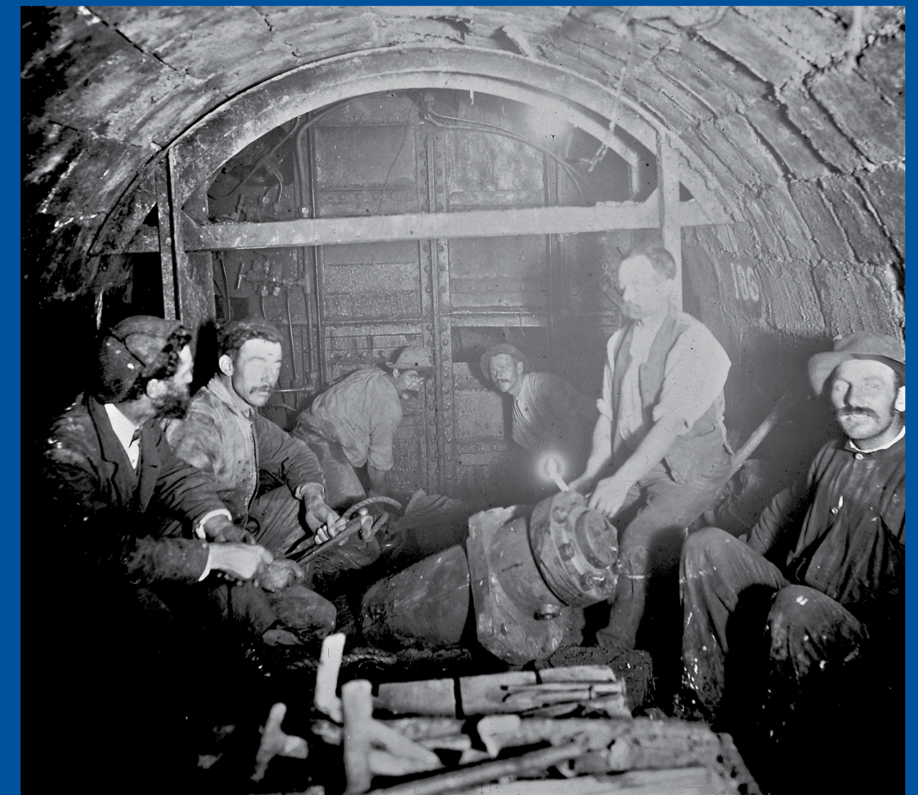
Tunnel shield in compressed air under Port Melbourne. Hobson's Bay Main - 1893
