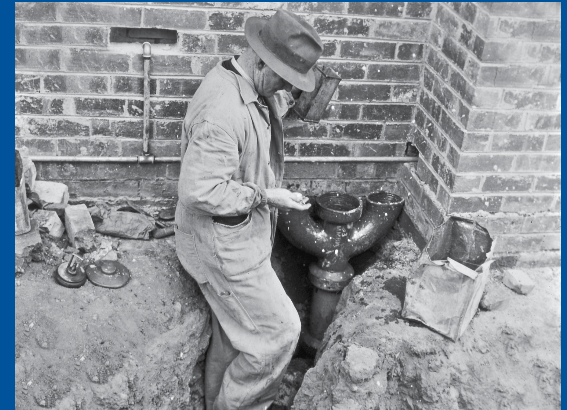
Inspector conducting hydrostatic testing on new house connections
